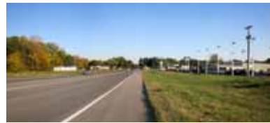
Existing view of Old US 31 looking east from the bypass interchange.
